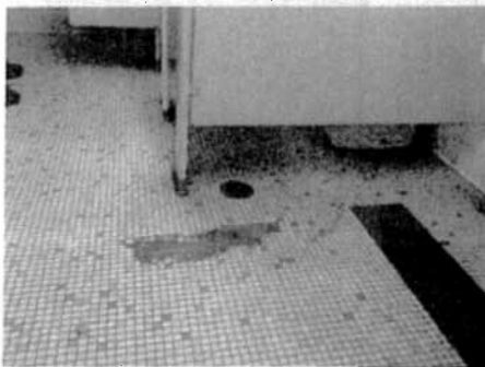
Damaged toilet room floor drain and tile.
